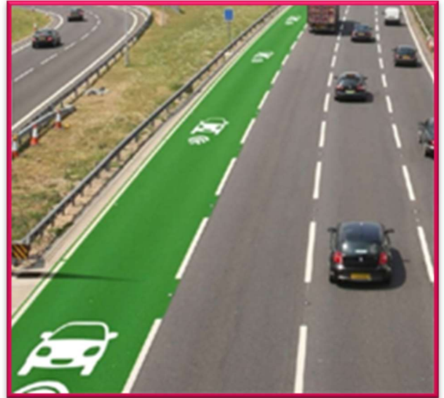
Figure 39: Wireless in road charging
